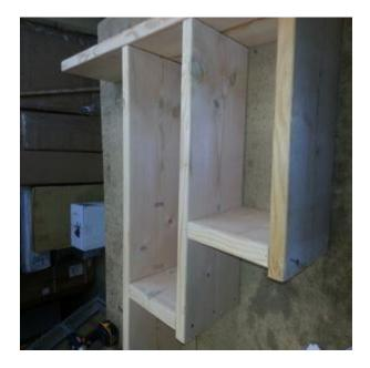
Place The 2" x 12" x 35-1/2" Under The 2" x 12" x 9-1/2". Screw Nice And Tight And Screw On Too The Size Of The 2" x 12" x 44" As Well.
